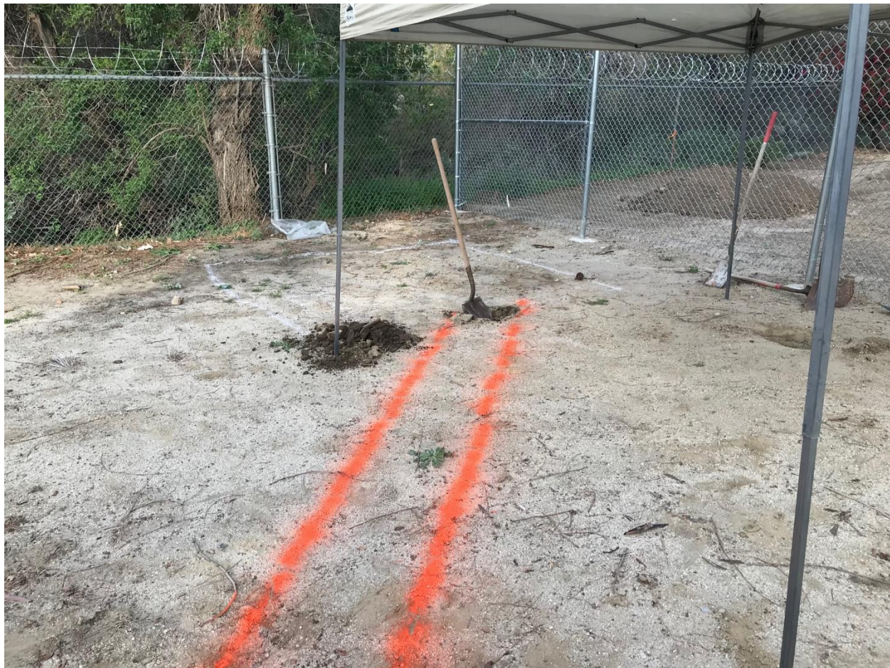
Figure 3: Marking of Trench Line for Conduit Run
