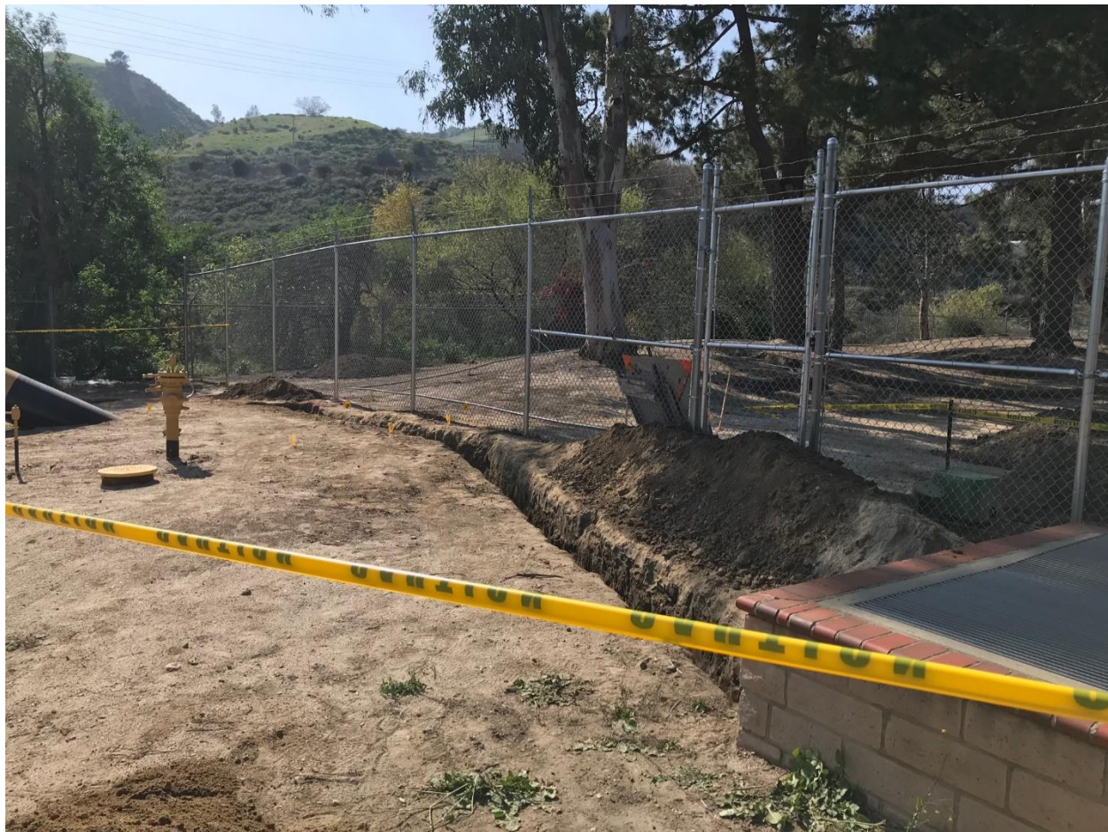
Figure 4: Trench for Conduit Run
