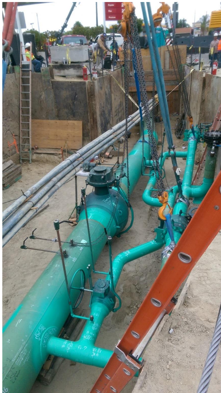
Figure 5: Cherry Site: New Bridle Assembly in Excavation Area
