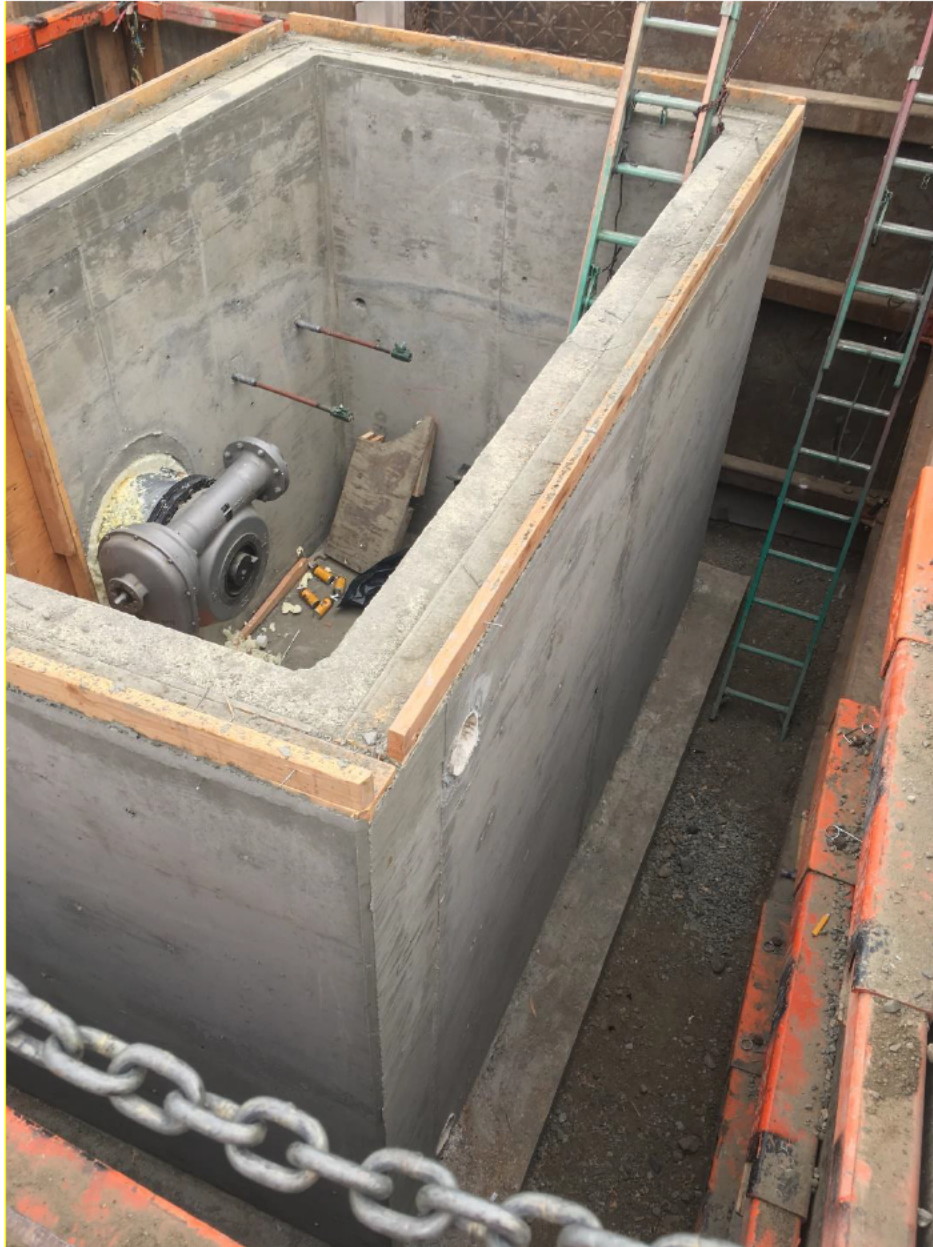
Figure 4: New Concrete Vault
