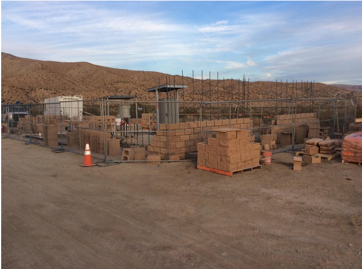
Figure 4: New Block Wall in the Foreground, New Canopies in the Background
