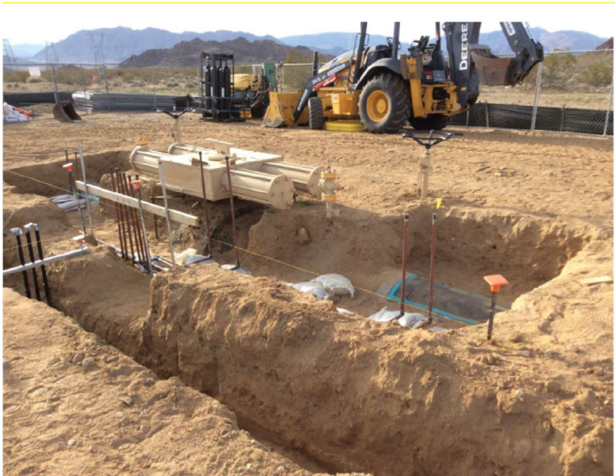
Figure 4: Excavation For New Sense Lines and Conduit
