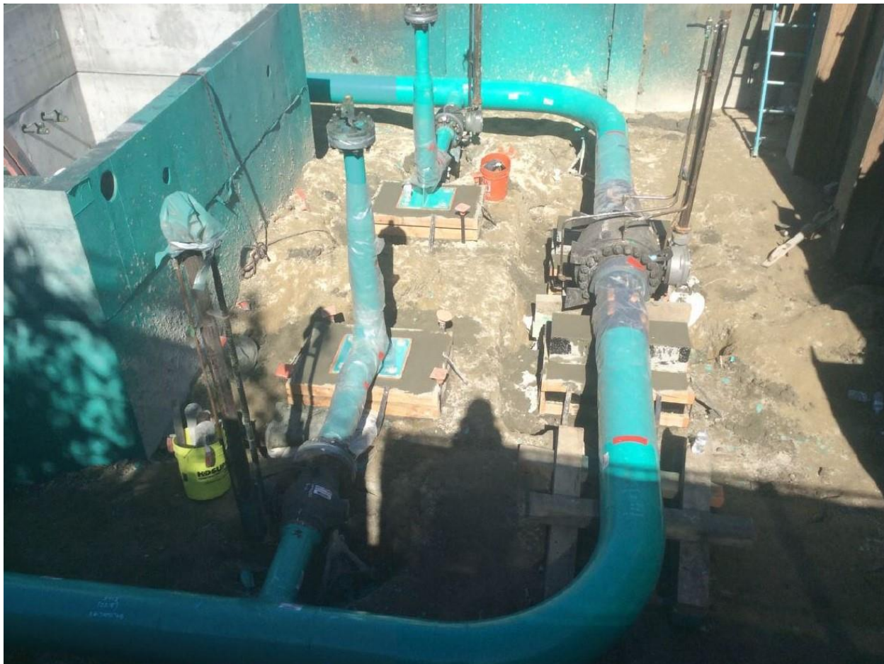
Figure 4: New Valve Assembly and Concrete Supports
