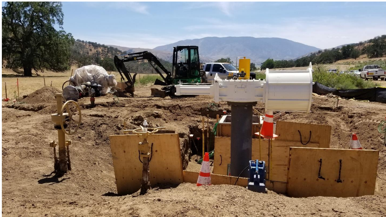
Figure 4: New Actuator and Excavation for Instrument Taps
