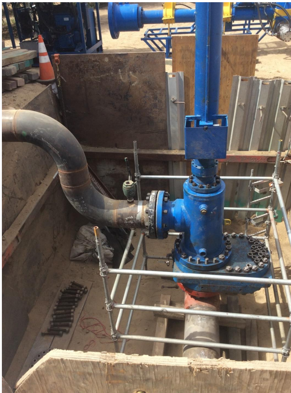
Figure 4: Stopple Fitting with Temporary Bypass
