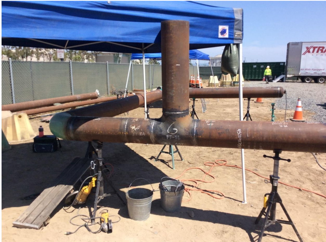
Figure 3: Fabrication of the New Blowdown Assembly
