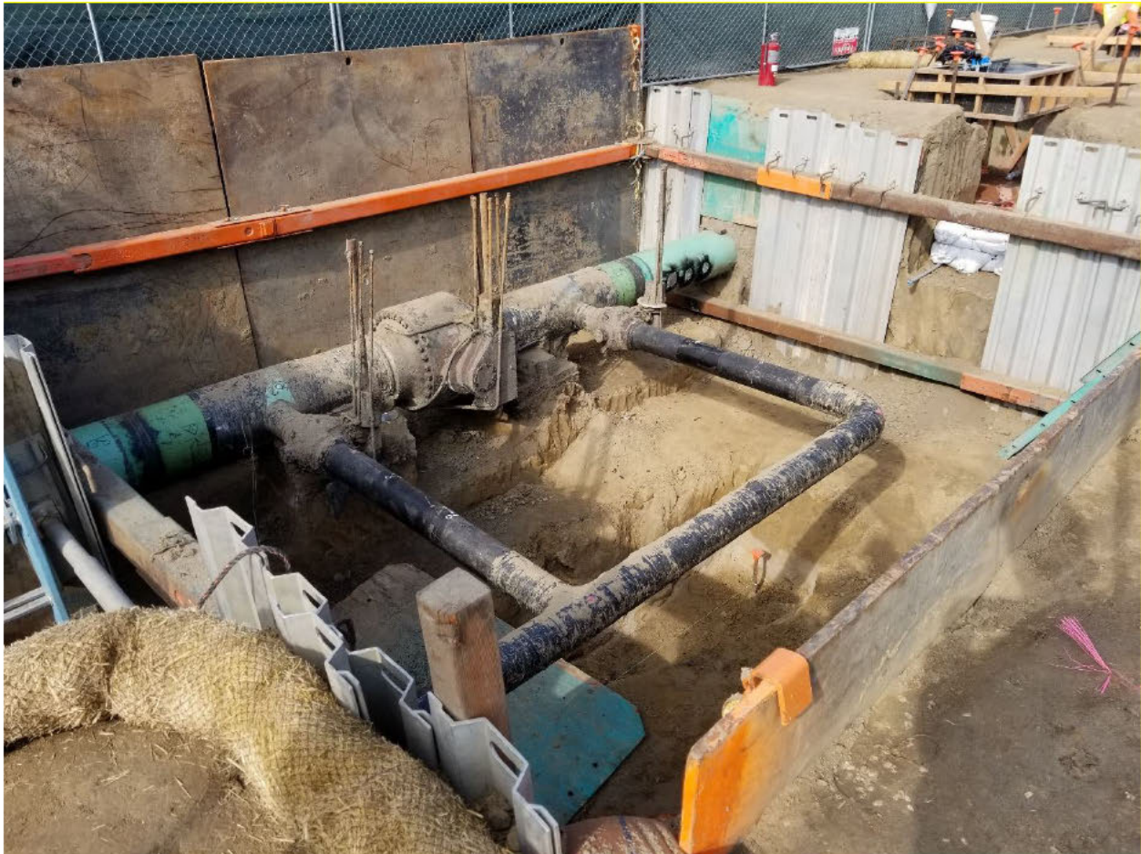
Figure 4: Excavation around Mainline Valve Assembly
