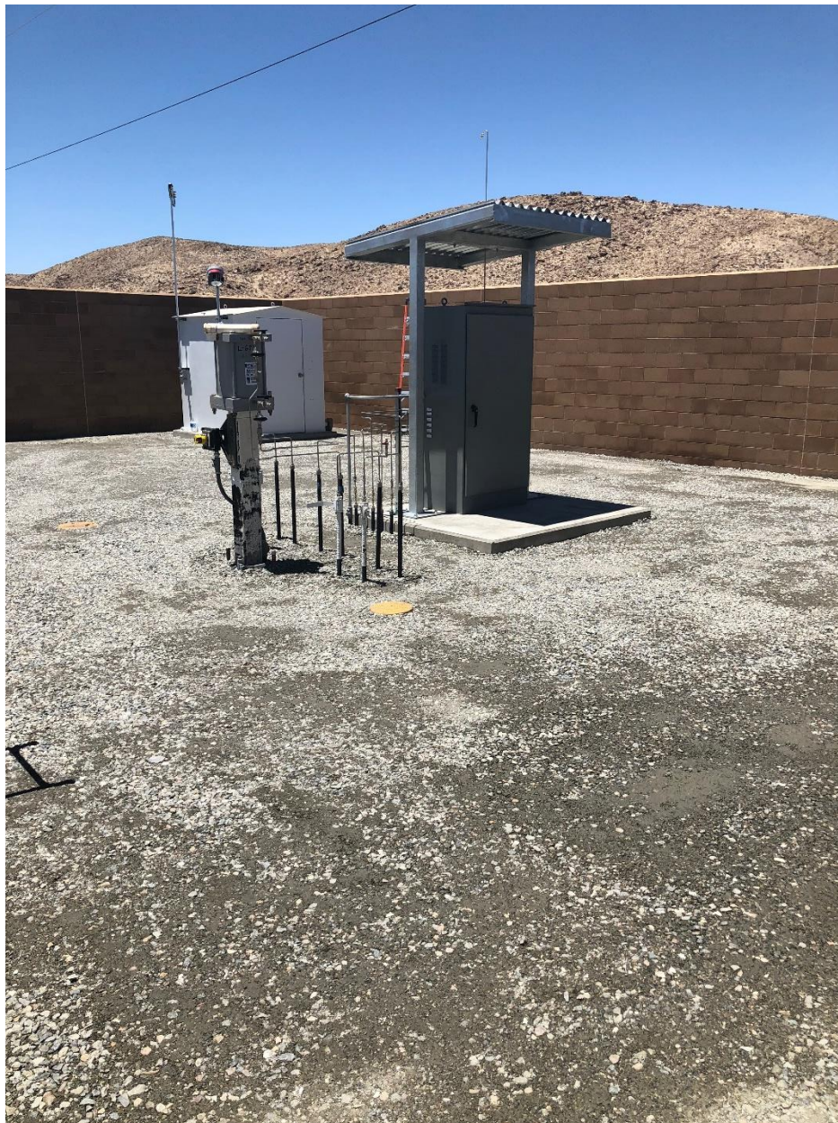
Figure 4: New Block Wall in Background, New Automation Equipment in Foreground
