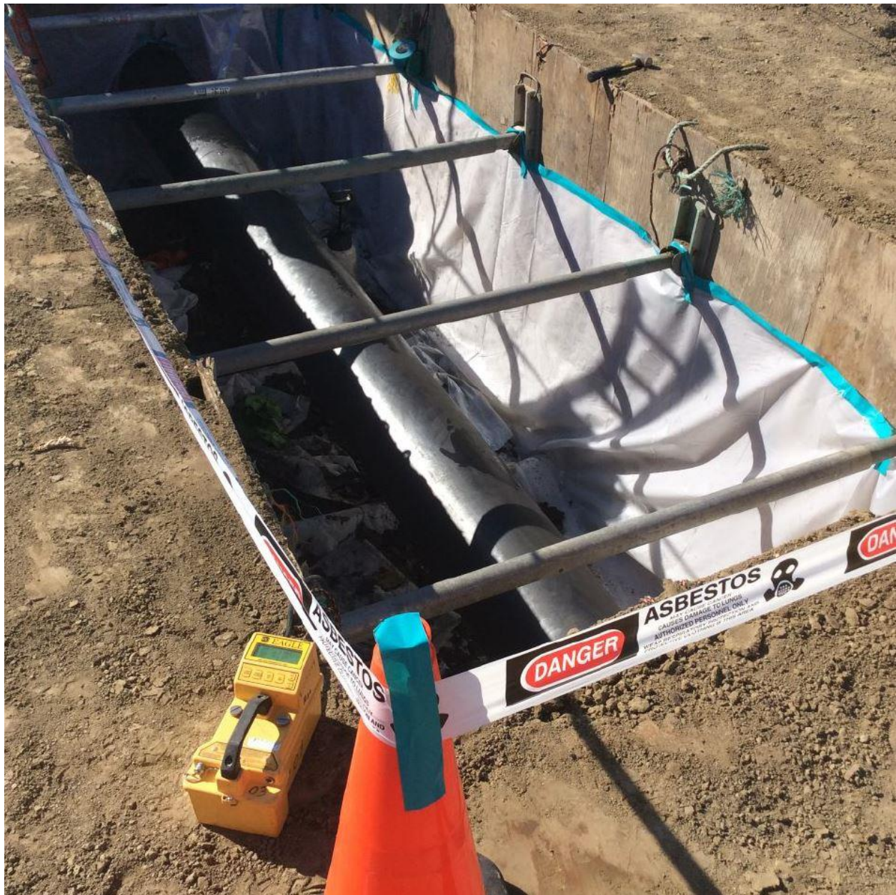
Figure 7: Abatement Activities at the Mills Station
