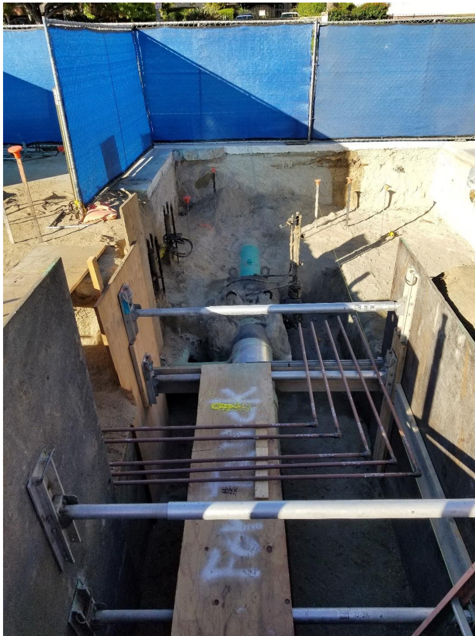
Figure 8: Mainline Valve Excavation and Instrument Piping
