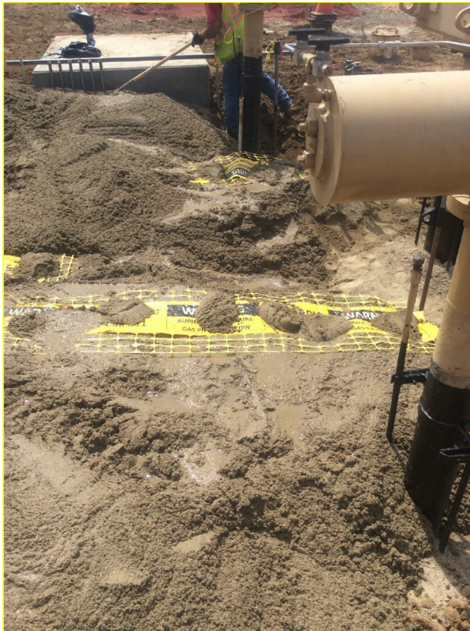
Figure 10: MLV 20.7 – New Actuator in Foreground, Trenching in Background
