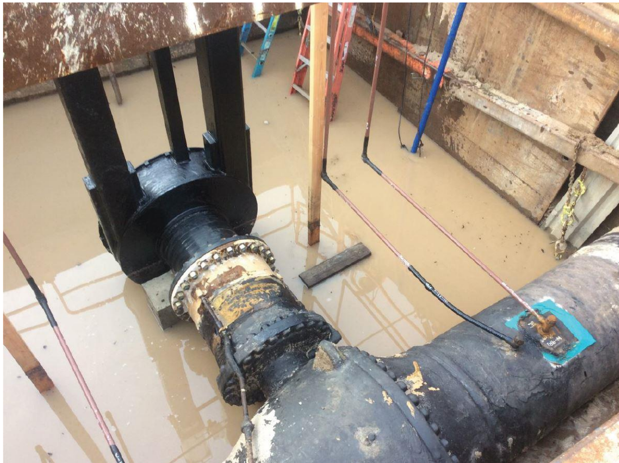
Figure 4: Dewatering of Excavation
