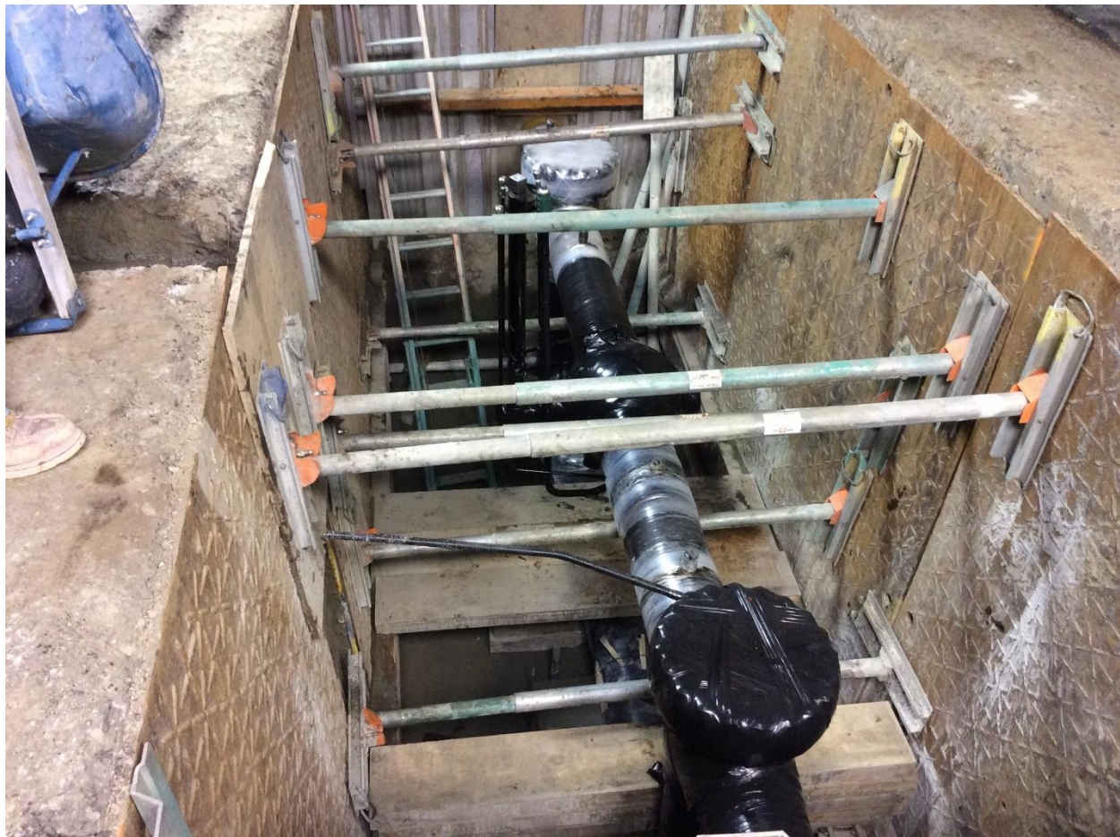
Figure 4: Excavation, New Check Valve and Two Stopple Fittings
