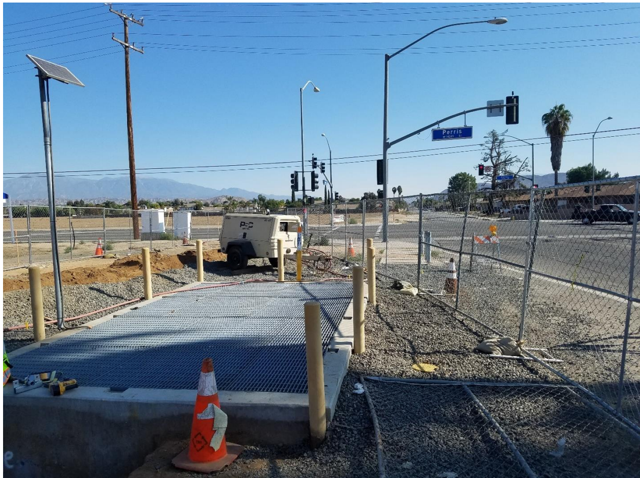
Figure 7: MLV 16 – Site With Temporary Fencing
